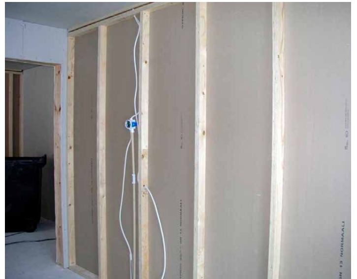
Figure 5. Kerto LVL studs in partition walls.
