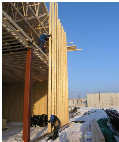
Figure 3. Kerto LVL studs in exterior walls.
