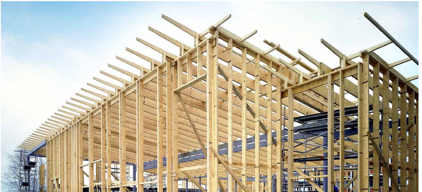
Figure 4. Kerto LVL as framework studs .
